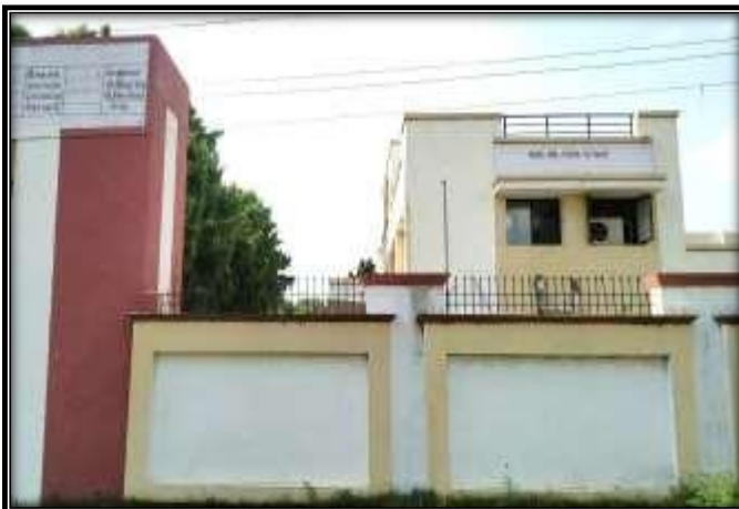
Figure 15 RO water treatment plant
