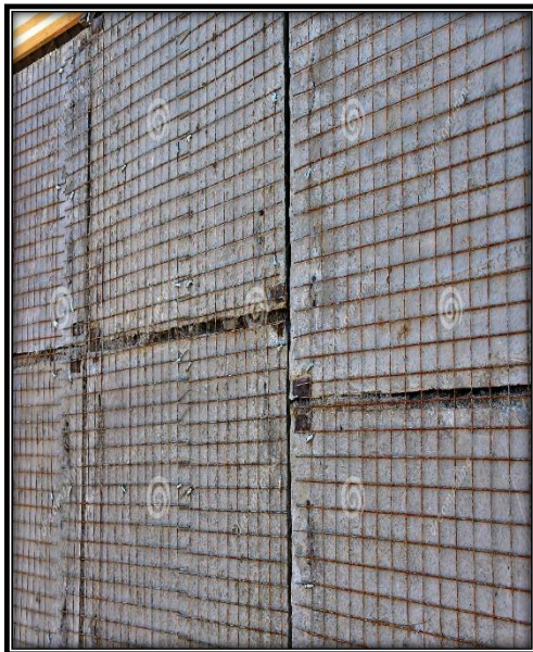
Figure 76 Wall Strengthening by Steel wire mesh
