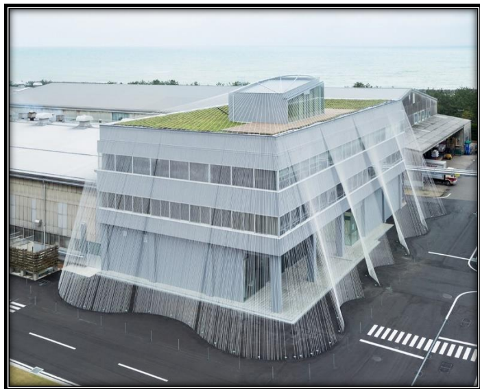
Figure 89 The Cabkoma Strand Rod
