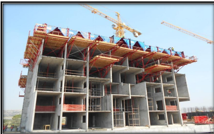
Figure 80 Tunnel Formwork System
