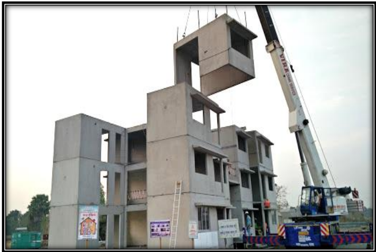
Figure 77 3D Volumetric Construction
