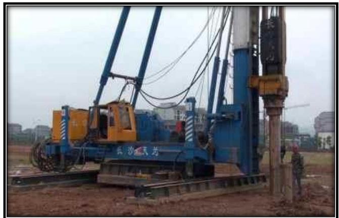
Figure 99 Pile driving Equipment
