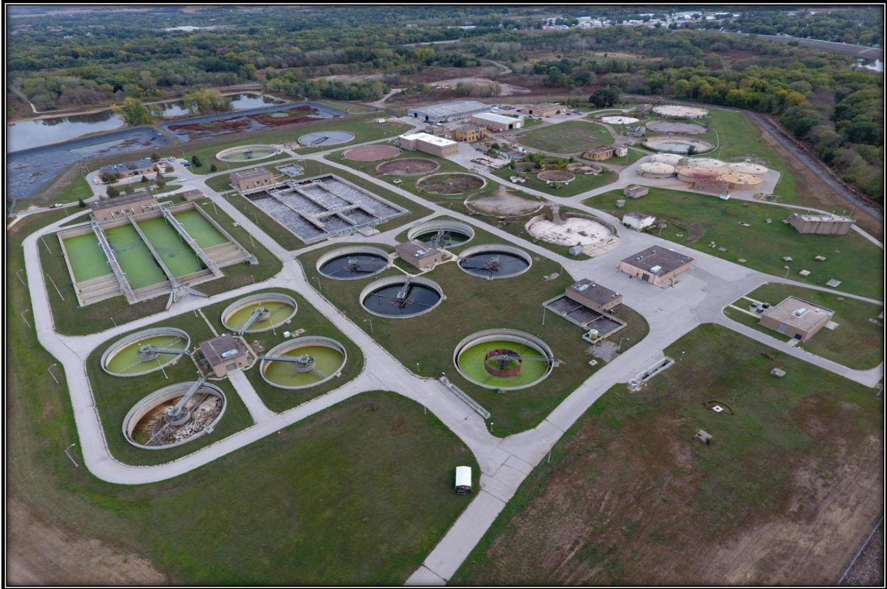
Figure 50 Sewage Treatment Plant
