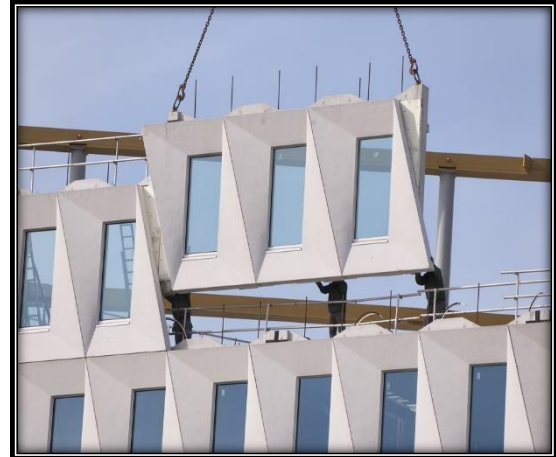
Figure 79 Precast Flat Panel Module
