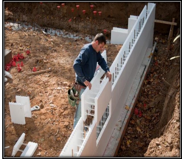
Figure 83 Insulating concrete formwork
