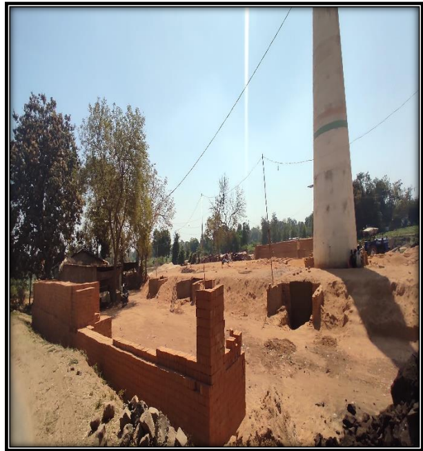
Figure 37 Brick Manufacturing Plant
