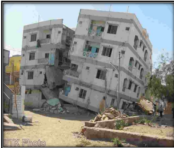
Figure 69 Collapse of RCC building during Bhuj earthquake 2001
