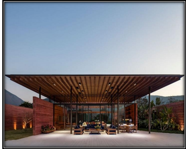
Figure 90 Residential house constructed by Pigmented concrete
