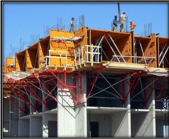
Figure 80 Tunnel Formwork System
