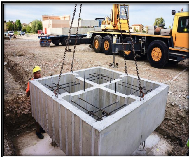
Figure 82 Precast Concrete Foundation
